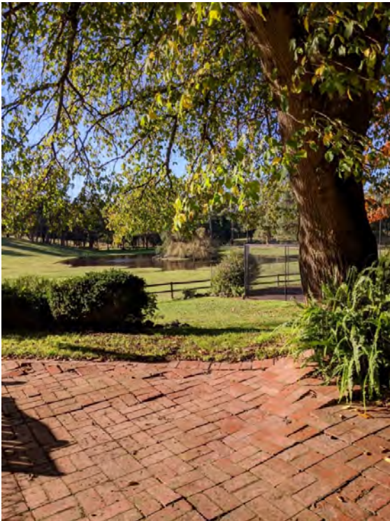
View to the dam
